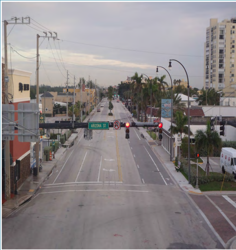
SR A1A looking north at Arizona St.
