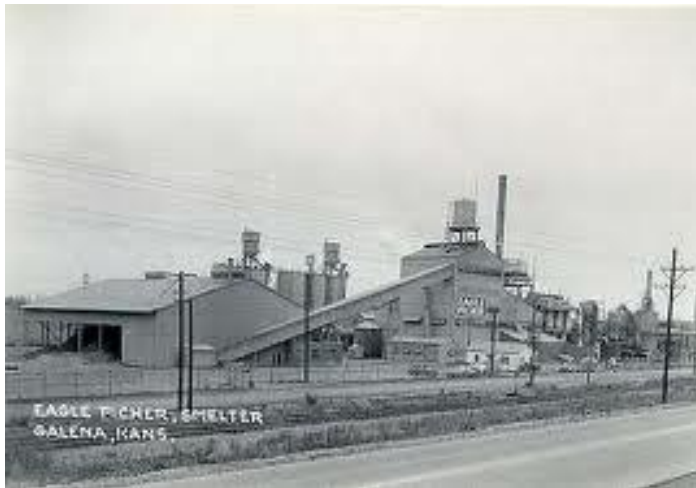
Smelter as shown during operating years.
