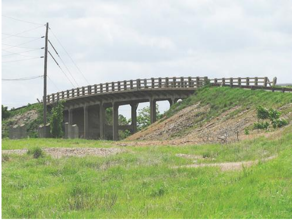
The Galena Viaduct
