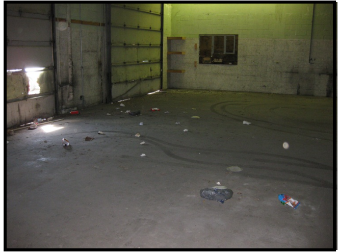
Photo: Two former hydraulic lifts were located in the maintenance area garage.
